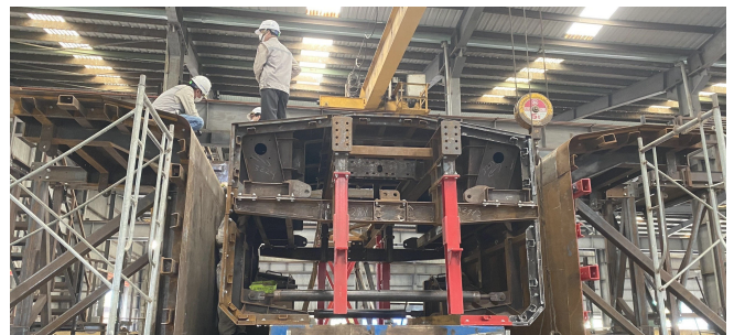
Moulds & Formwork travelers
