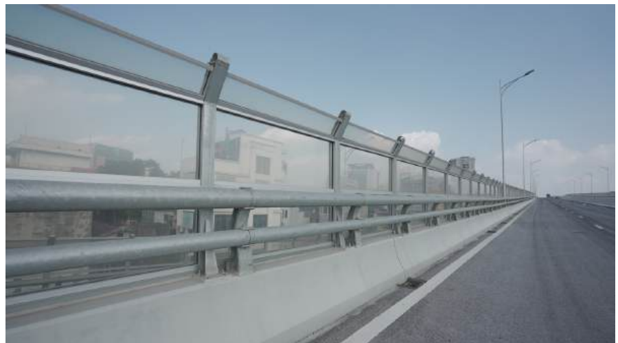
2. Hanoi's city elevated ring road No.2
