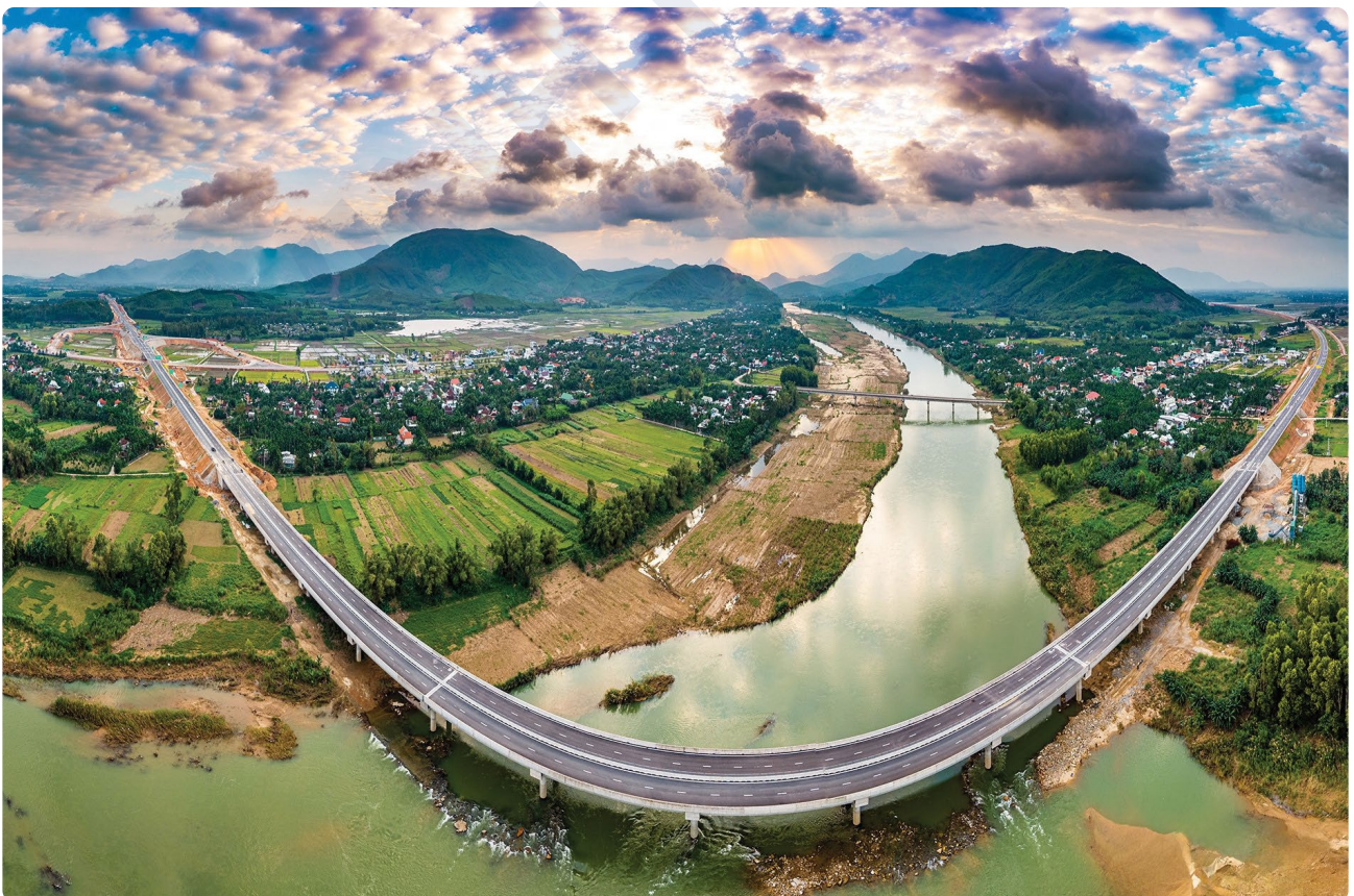
VHF Finger Expansion Joints have been installed along the entire Quang Ngai – Hoai Nhon Expressway (Vietnam)
