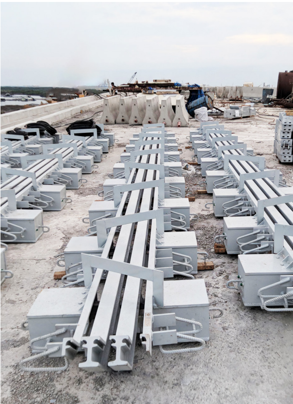
Installation VHM modular expansion joints in Mo Nhat bridge project (Ba Ria - Vung Tau)
